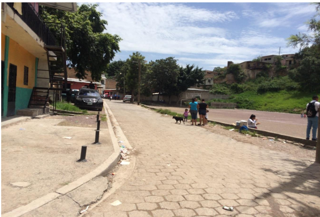
Adoquín a desmontar
