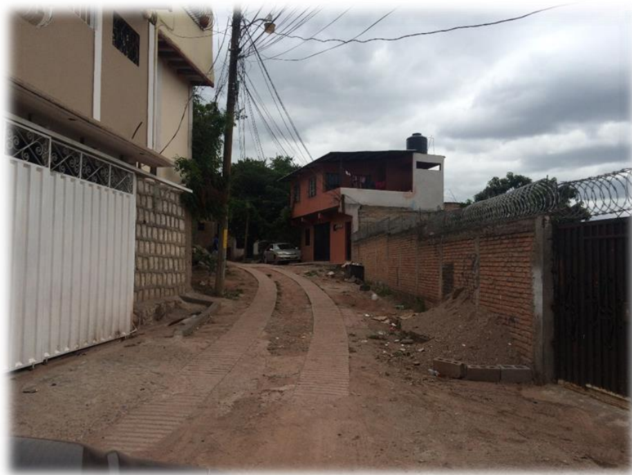
HUELLAS VEHICULARES A DEMOLER
