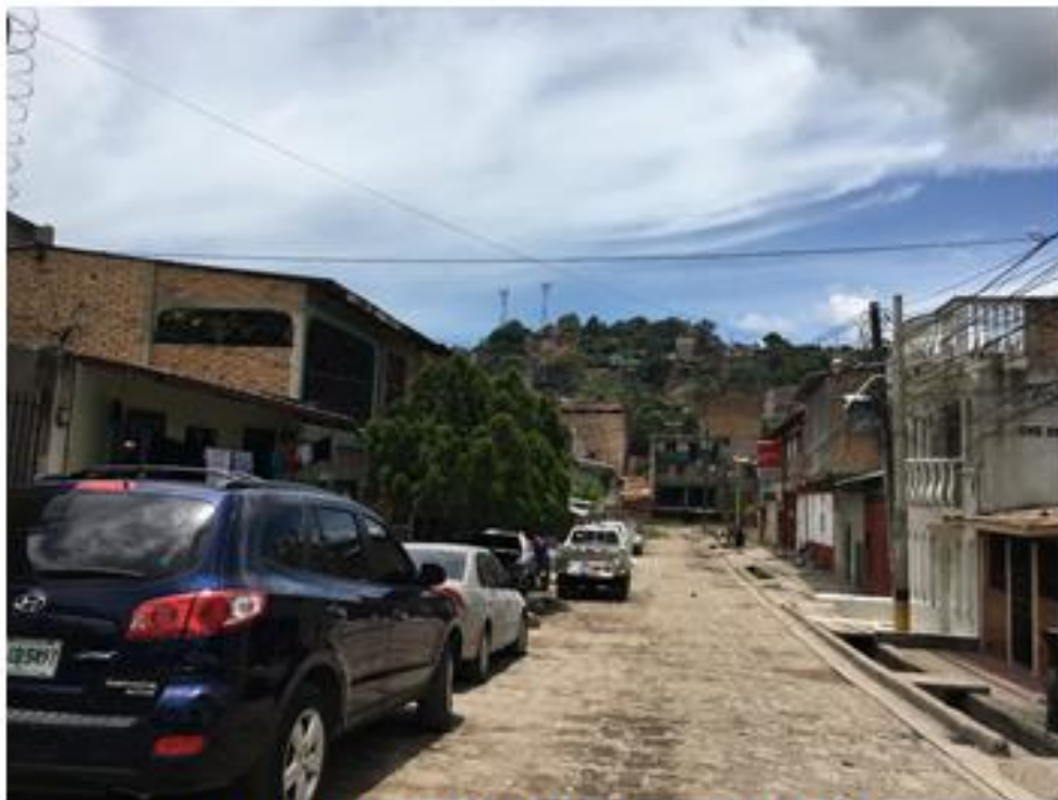
FINAL DE WHITE TOPPING. TRAMO C.
